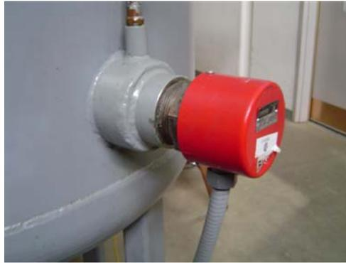
Figure 21. Heater attached to the tank to maintain temperature
